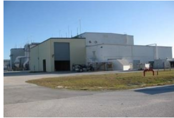
CCAFS Upgrades Hangar AM, Cape Canaveral Air Force Station, FL
