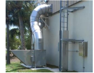
Repair Rooftop Exhaust, Chem Lab - Cape Canaveral Air Force Station, FL
