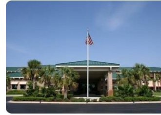
USDA Remodel of General Purpose Shed, USDA Eaves Painting, USDA Site Work and Non-Skid Paint at Shed and Ramp - Ft. Pierce, FL
